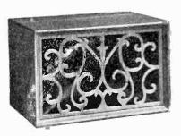
Material of Horn-Hard Rubber: Finish-Mahogany, Type of Magnet-Half Ring; Action -Electro Magnetic; Dim.-147 x 9% x 916; (Horn is of Molded Construction providing 271/2 in, of air column); Solid Mahogany Cabinet; Price-\$30.00,
