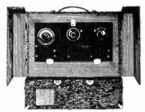
Trade Name-"Porto-O-Radio"; Type-Tuned Radio Frequency; Tubes-6; Battery-"A" Dry; "B" 90 Volts; Controls-1; Tuning, 1; Antenna -None; Dim.-16 x 16 x 4; Weight-24 lbs.; Style-Portable; Price-\$170.00.
