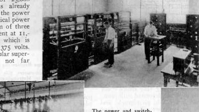
The power and switching equipment of the superpower broadcasting station at WGY is shown at the left. This station has been on the air with 50,000 watts under an experimental license issued by the Department of Commerce
